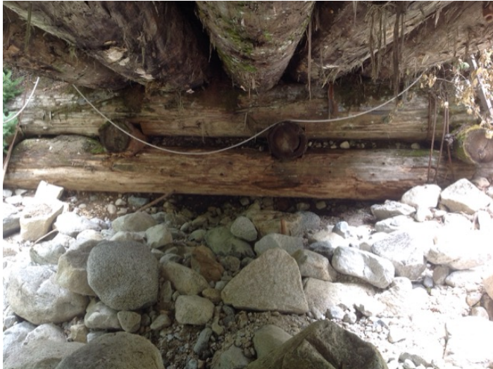
Right Bank Abutment when facing downstream
