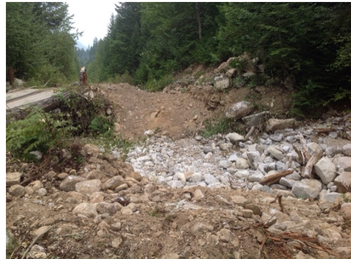
machine bypass just upstream
