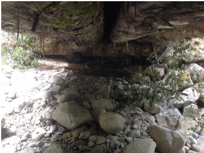
Left Bank Abutment when facing downstream
